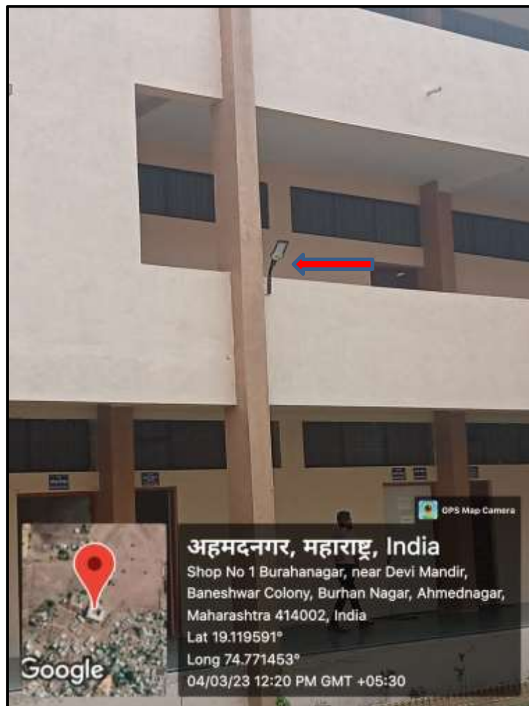
Use of LED and Energy efficient equipment
