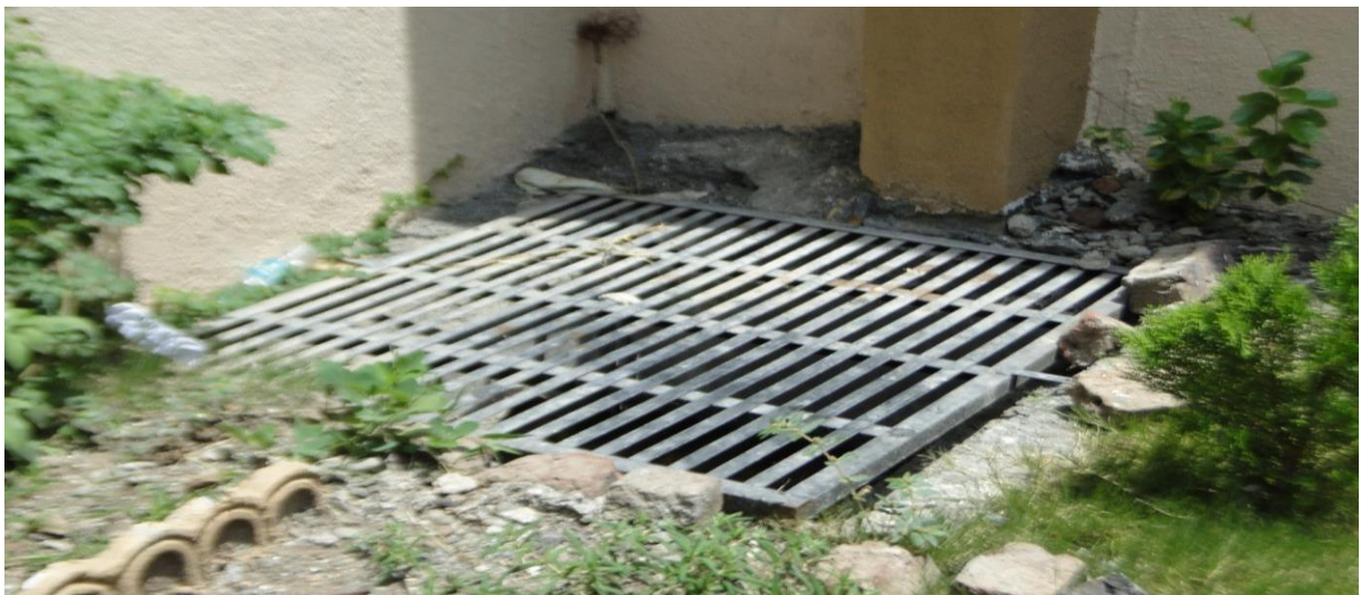
Rainwater Deposited Pit
