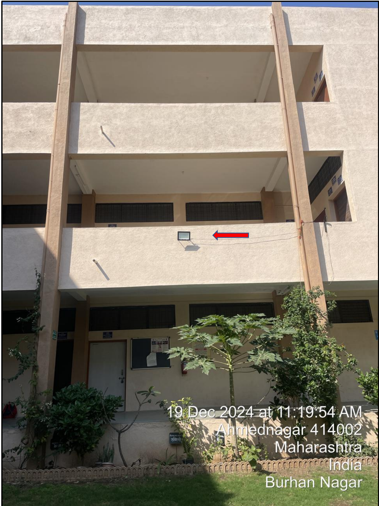
Use of LED and Energy efficient equipment
