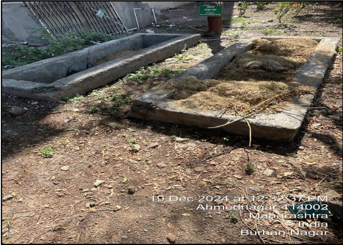
Varmi compost for waste recycling system
