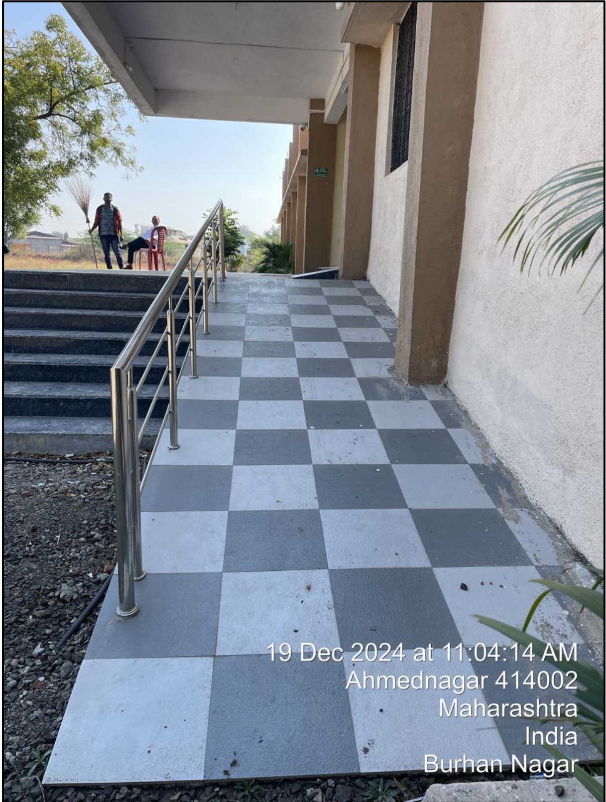
Built Environment with ramps/lifts for easy access to classrooms.
